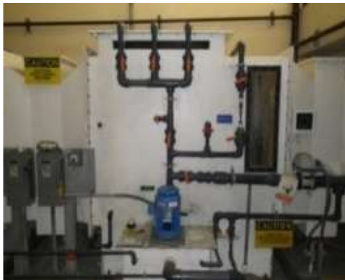
Solids Handling Building odor control scrubber
