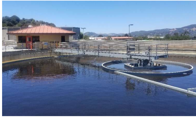
Secondary clarifier in operation
