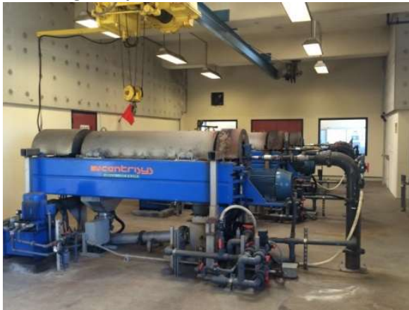
Existing Centrifuges
