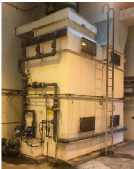
Headworks odor control scrubber
