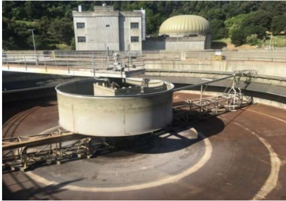
Secondary clarifier internal equipment
